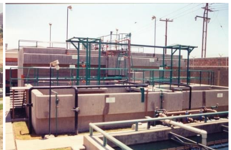
WWTP general view
