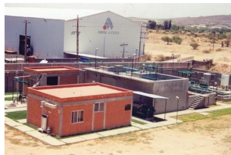
WWTP general view
